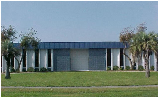
Trion Florida – On Site Machine Shop
